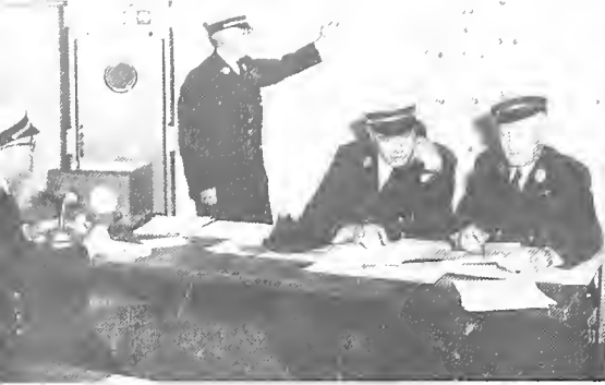
Fire communications room at the Control Center of the Boston Department of Civil Defense during a test exercise.
